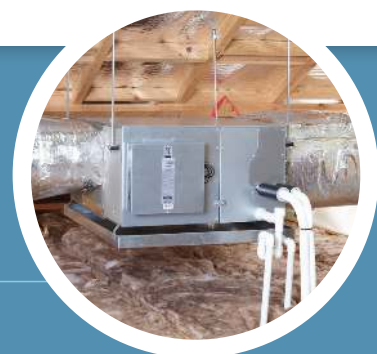
Indoor Fan Coil Unit installed within a roof space
